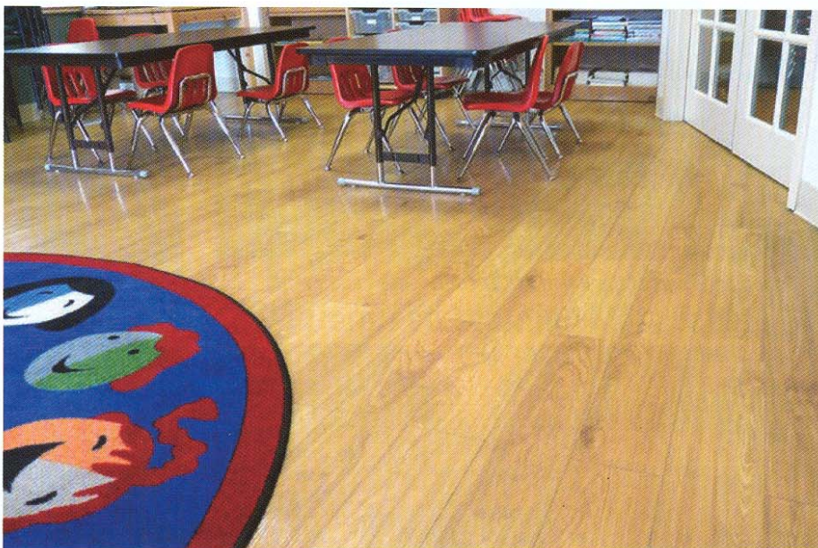
Vinyl wood plank floors convey a warm natural look, but are more durable than residential quality wood grain laminate.
